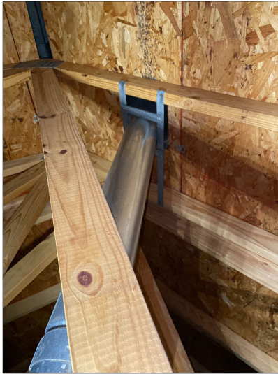
Furnace flue
