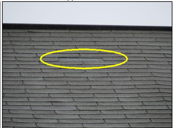
Broken/missing shingle
