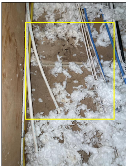
Stained drywall/hallway ceiling
