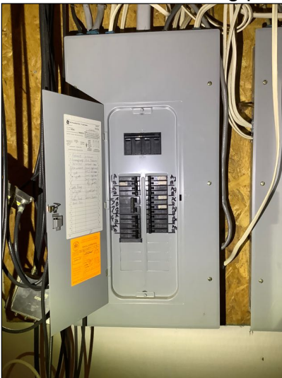
Unsecured wires entering panel
