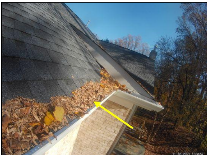
Debris noted in gutters. Recommend cleaning gutters so that water can properly drain.
