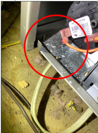
The air handler is dirty and appears to have a bio growth (mold like substance), we recommend testing for mold.
