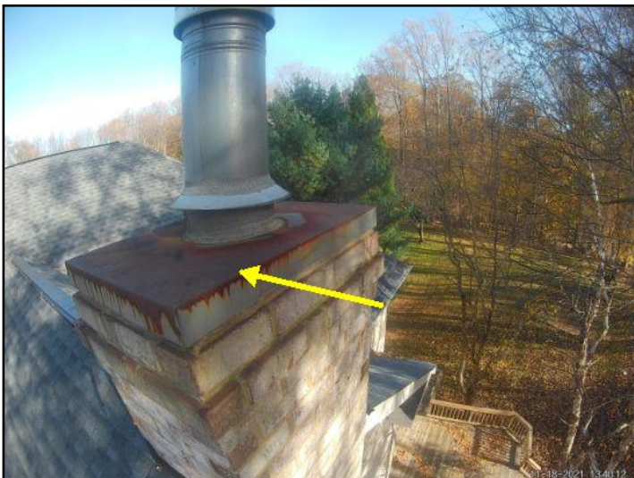
Chimney rain cap is severely rusted/deteriorated. Recommend painting to preserve its remaining life.
