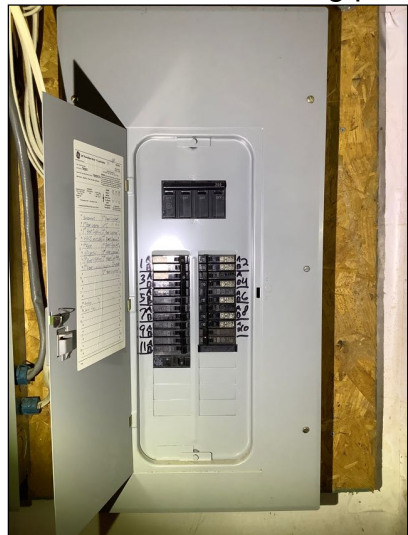
Unsecured wires entering panel
