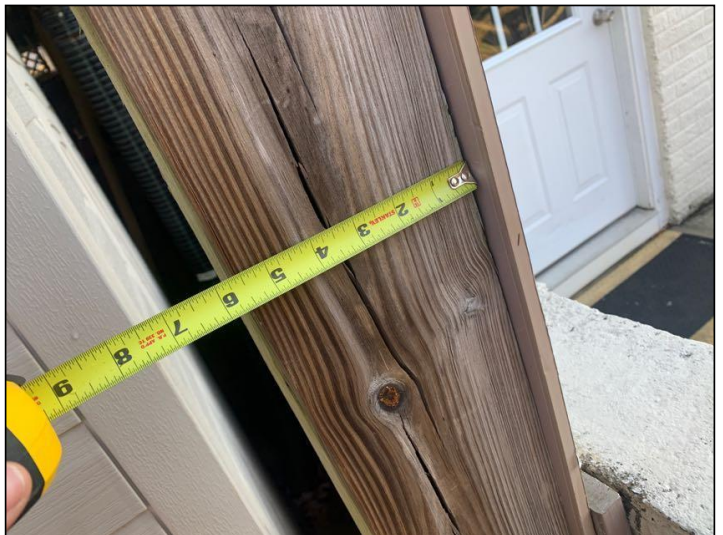
4x6 post noted supporting deck
