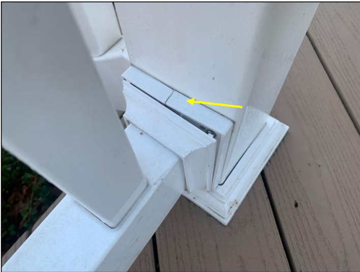
Cracked railing
