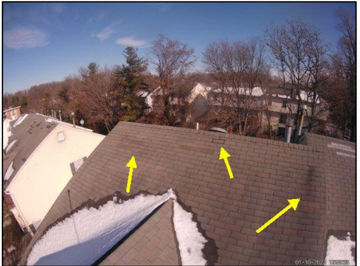
Repairs and stained/weathered shingles noted throughout roof
