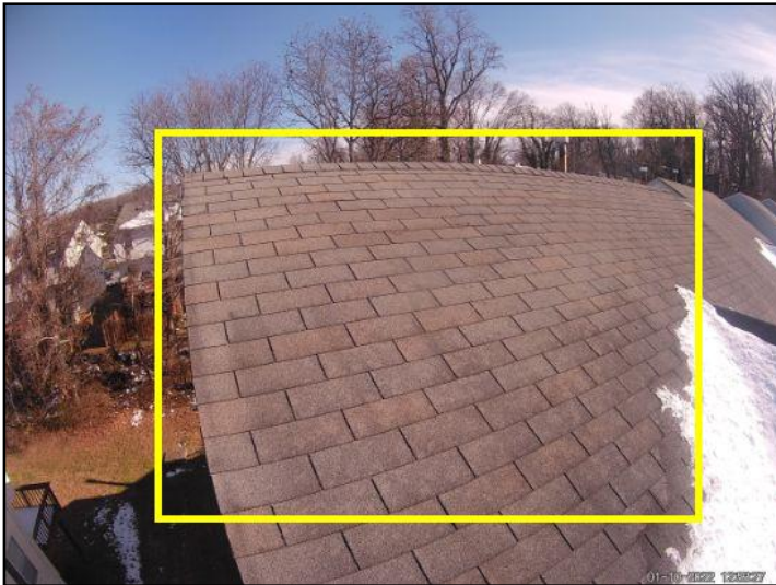
Aged/weathered shingles noted throughout
