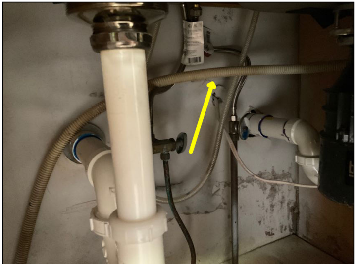
No high drain loop
