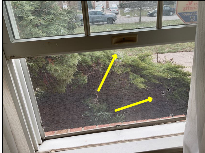
Screen damaged
