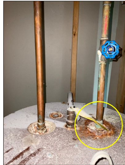
Corrosion (noted)
