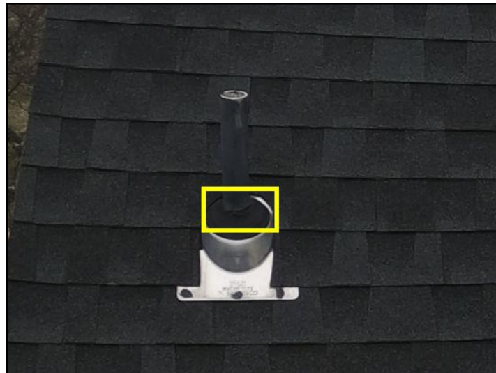
Deteriorated collar
