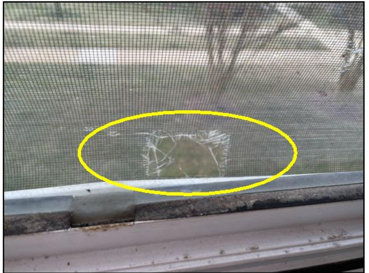
Damaged screen
