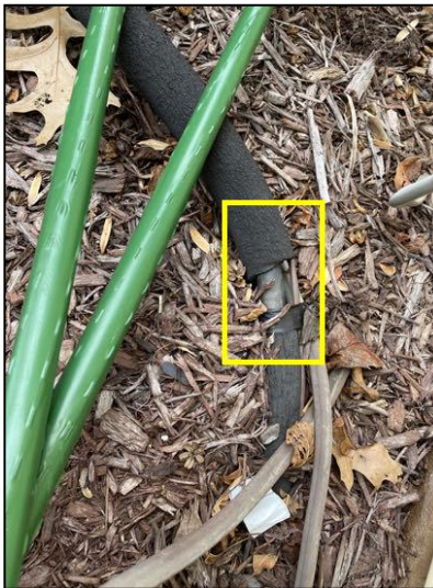
Missing insulation
