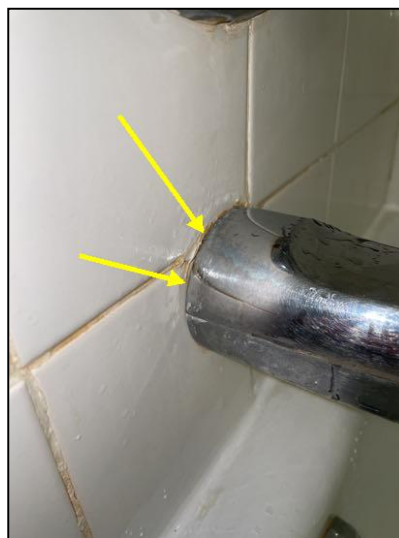
Deteriorated caulk
