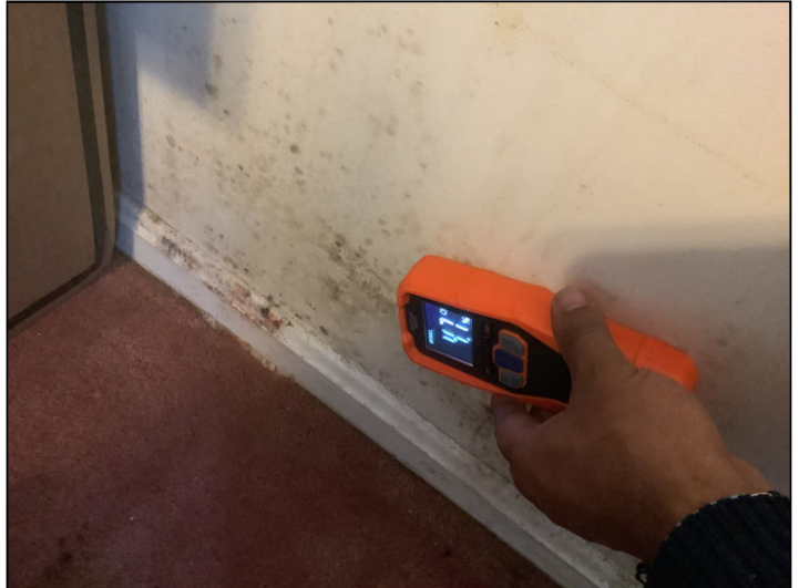
Tested dry at the time of the inspection.
