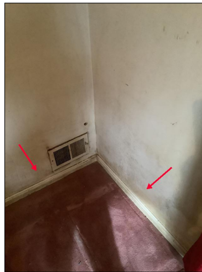
Areas tested dry at the time of the inspection.
