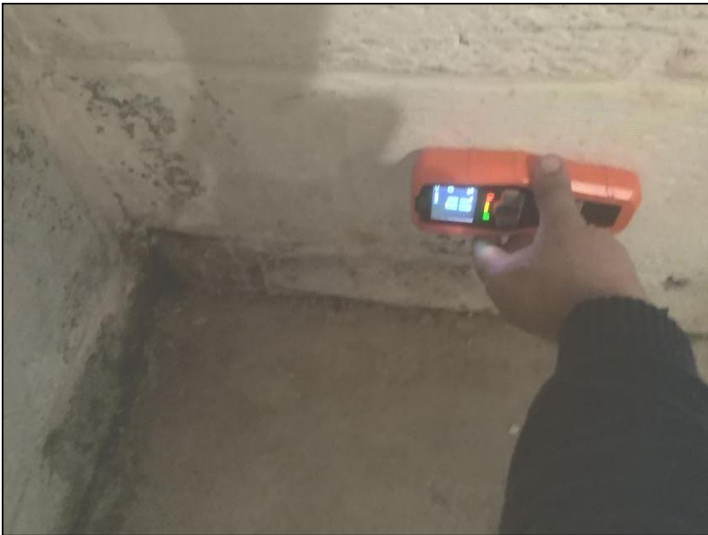
High moisture readings
